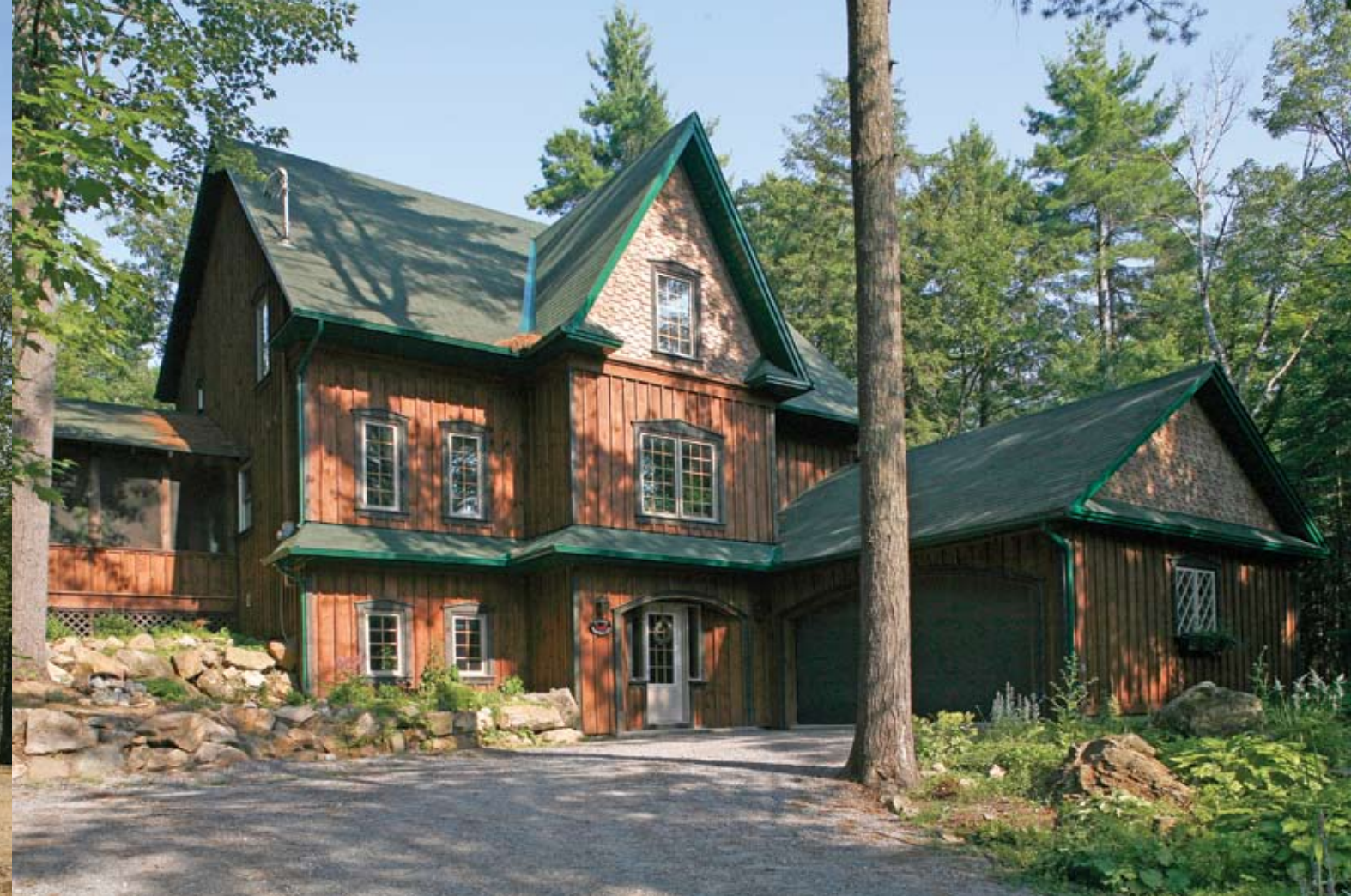
Peter Markhauser is careful to place the house on the lot in such a way that it almost seems to have grown there. The exterior board and batten, cedar shakes, and green roof and trim are simply elements drawn from the forest they inhabit. Graceful arches above the garage-door entry and the front door are designed to echo the curve of the barrel-vaulted ceiling inside
